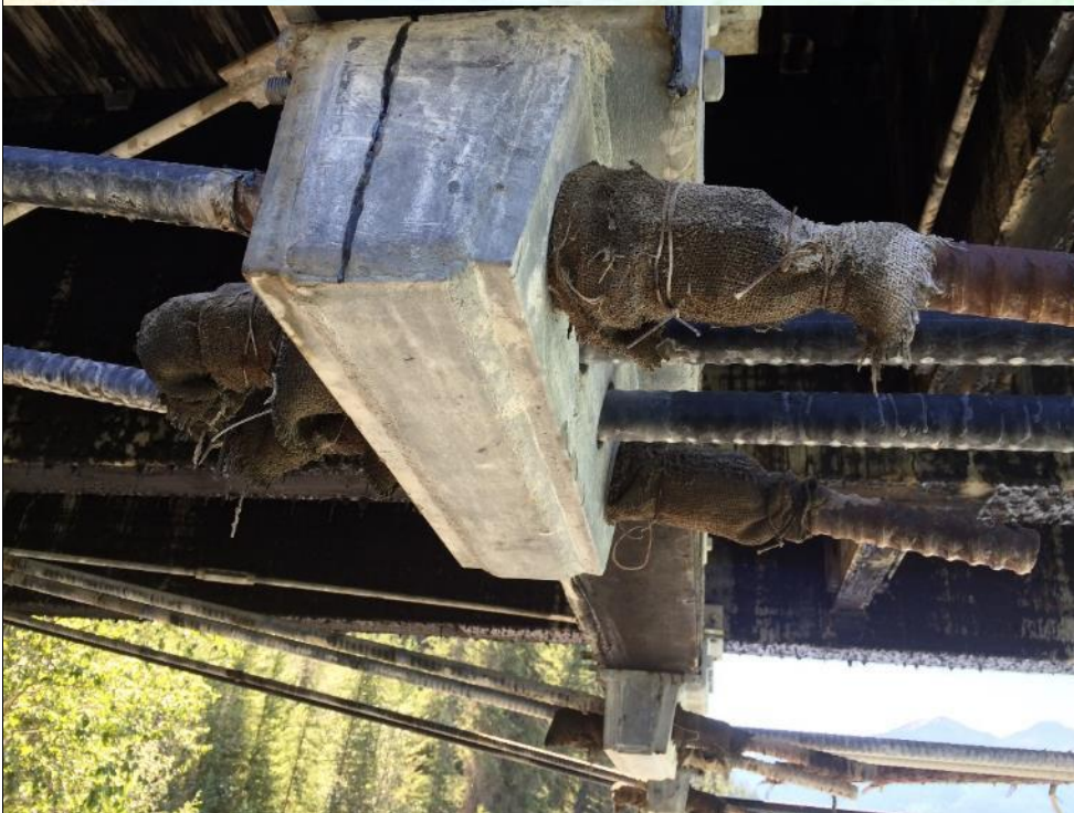
Photo #30 Span 2 bolstering bracket
