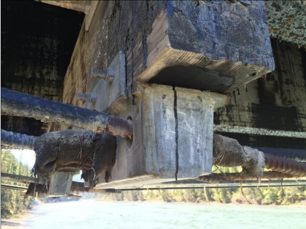
Photo #29 Span 2 bolstering bracket
