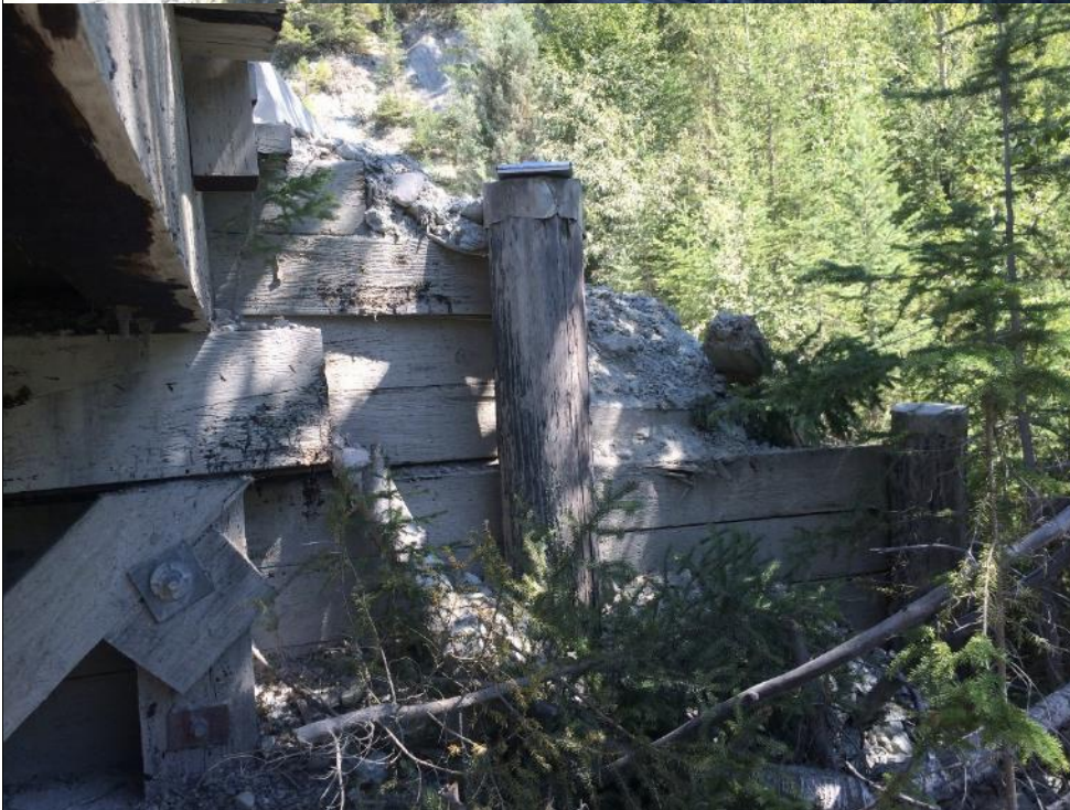
Photo #8 Abutment 1 D.S wingwall
