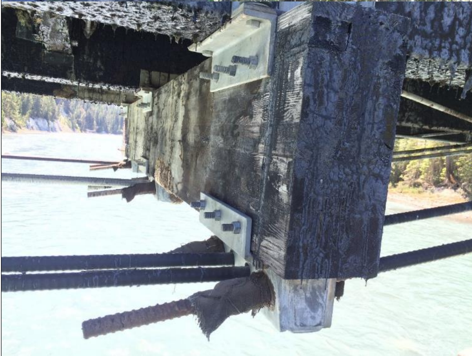
Photo #32 Span 1 bolstering bracket 2
