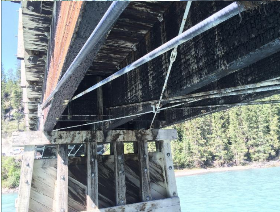
Photo #28 Underside of Span 2 looking to Abutment 2
