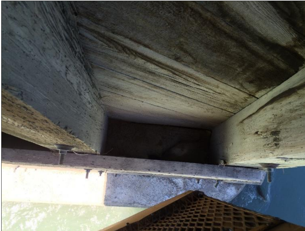
Photo #17 Pier 3 - looking downwards between shafts and behind sheathing
