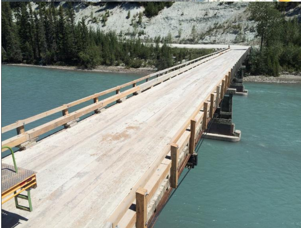
Photo #36 Top of deck, looking to Abutment 1
