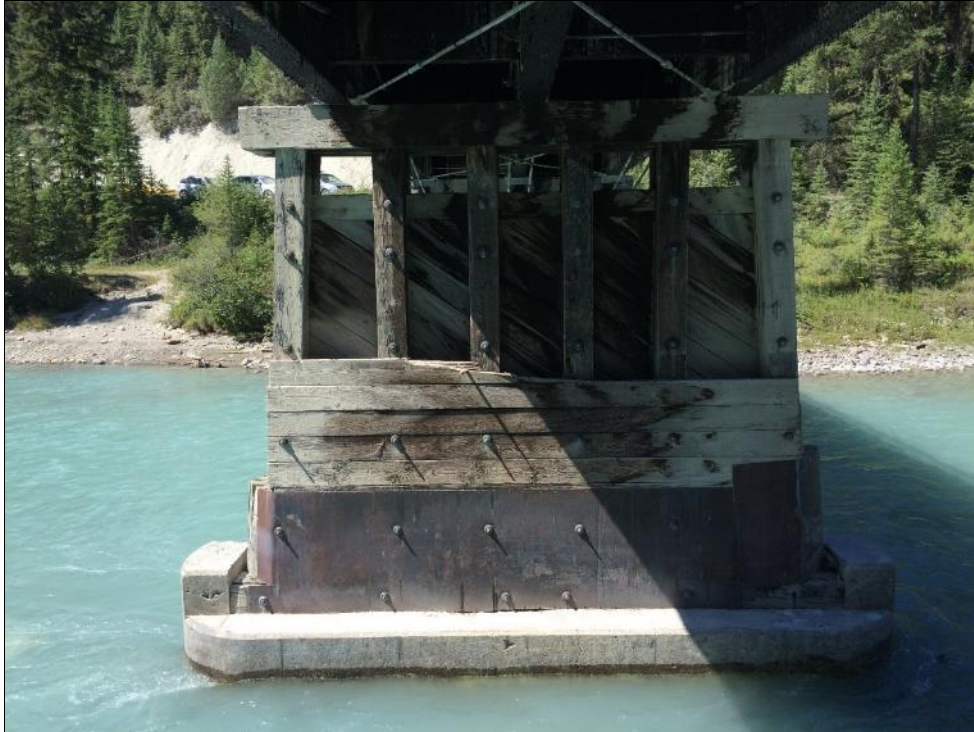
Photo #15 Pier 3 – looking to Abutment 2
