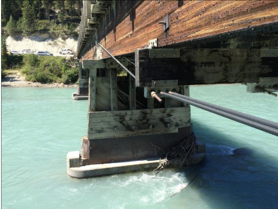
Photo #33 Span 2, Girder 1, bolstering bracket 2, looking to Abutment 2
