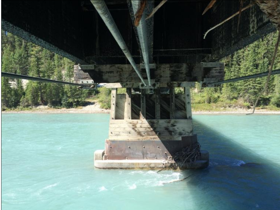
Photo #11 Pier 2 - looking to Abutment 2
