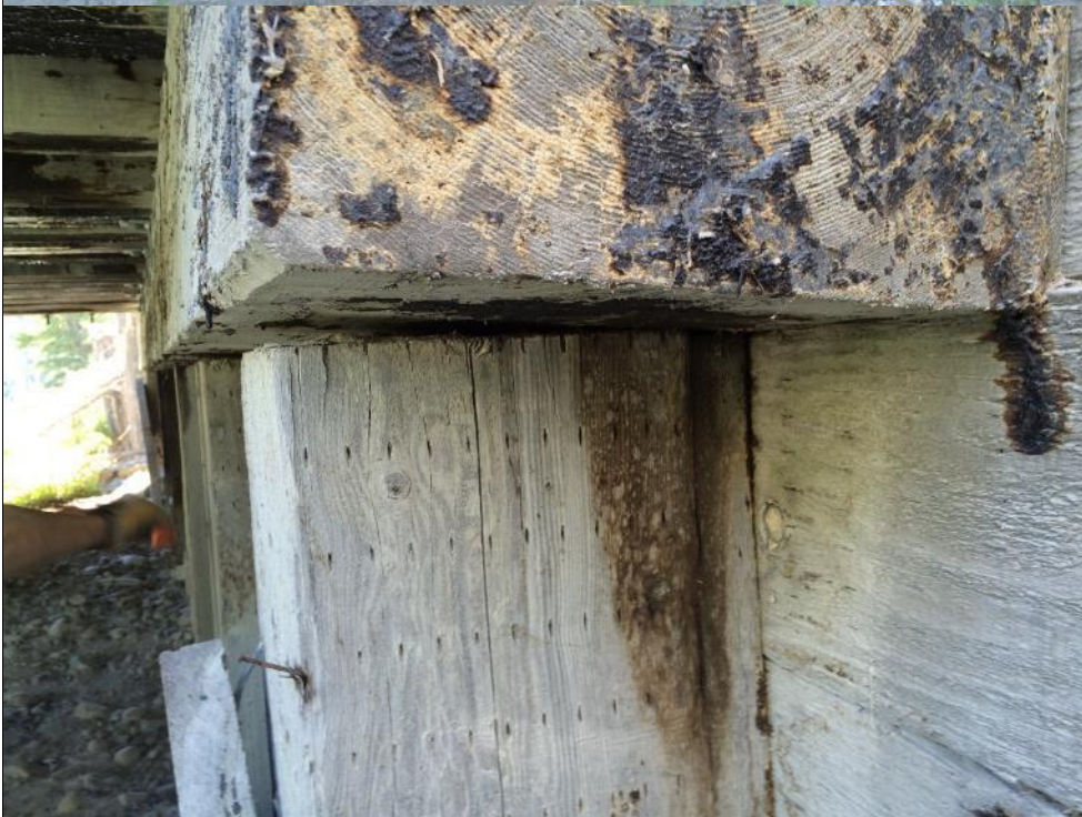
Photo #24 Abutment 2 - piles and pile cap
