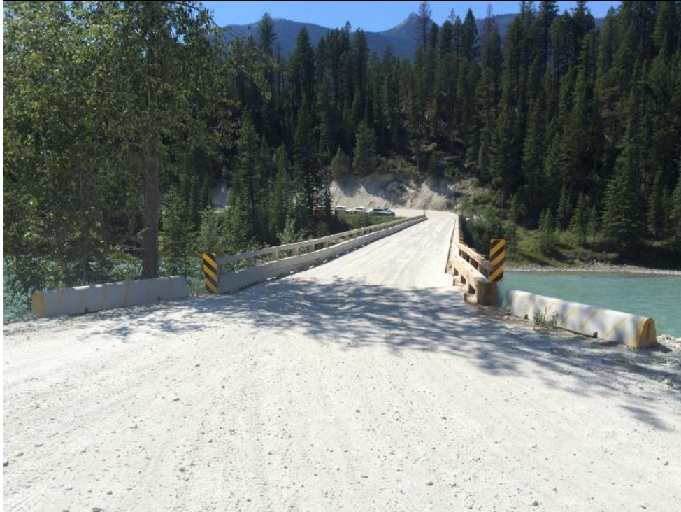
Photo #3 Abutment 1 (woods) approach
