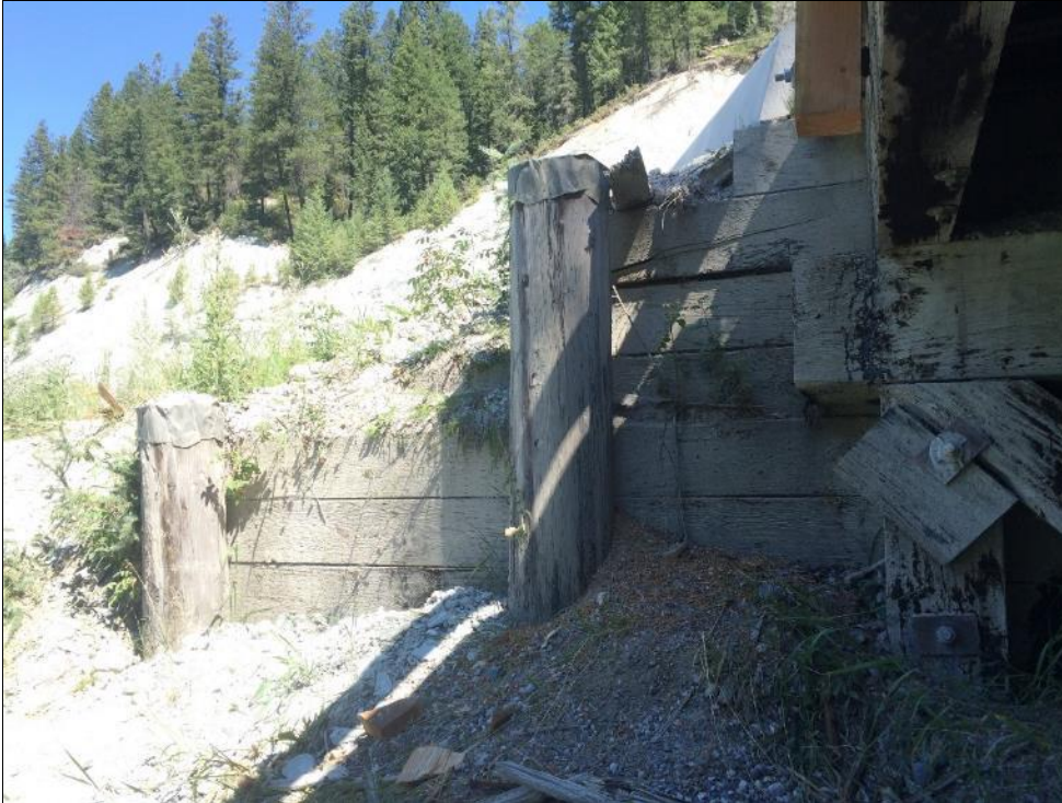
Photo #7 Abutment 1 U.S Wingwall
