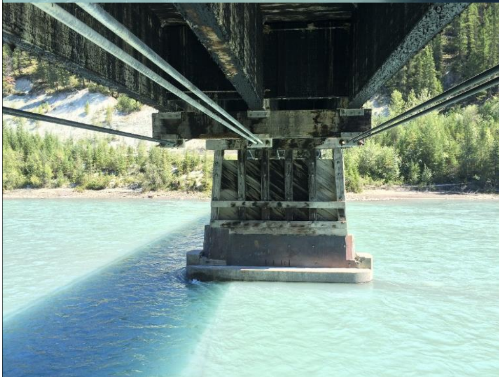
Photo #16 Pier 3 – looking to Abutment 1
