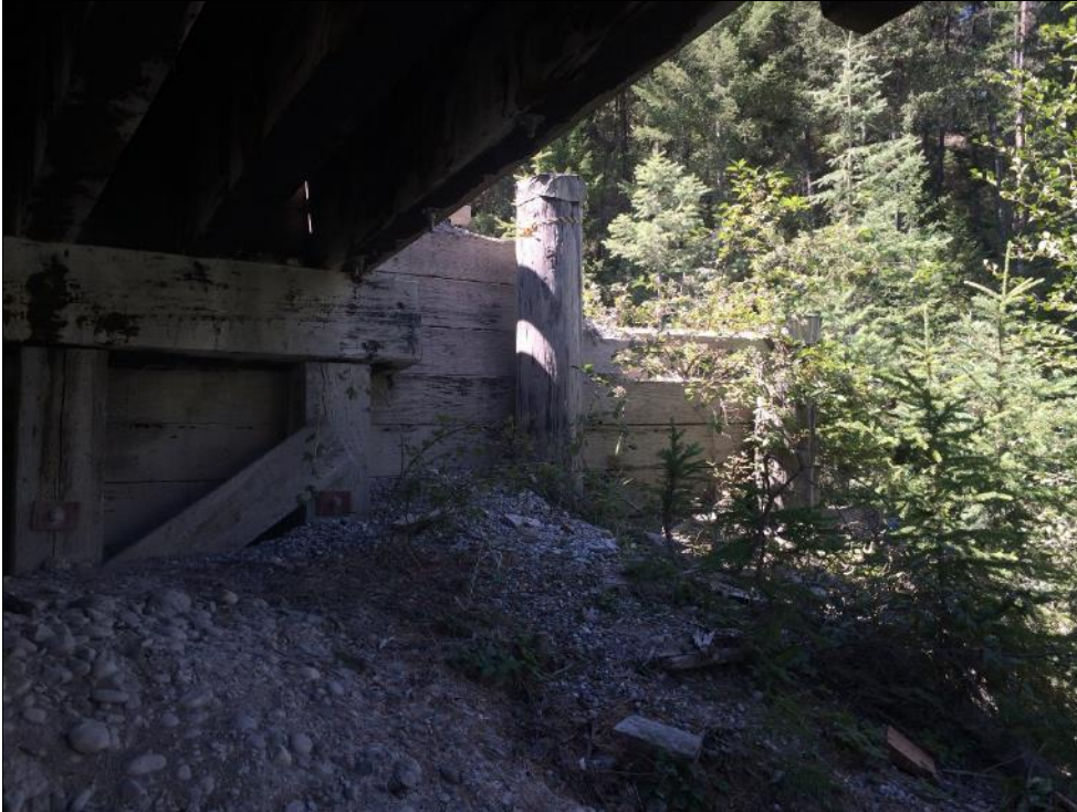
Photo #25 Abutment 2 - U.S wingwall
