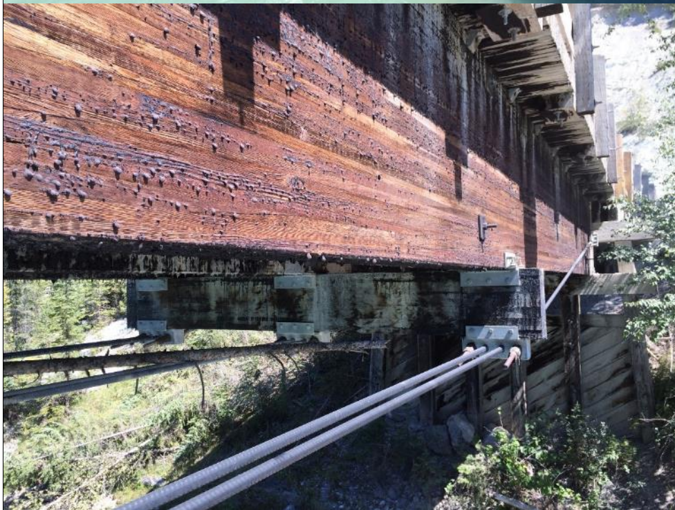
Photo #34 Span 2, Girder 3, bolstering bracket 1, looking to Abutment 1
