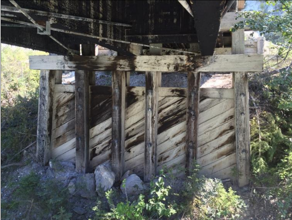
Photo #9 Pier 1 – looking to Abutment 1
