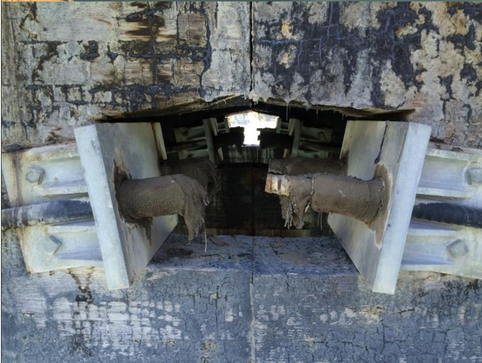
Photo #14 Anchorages of bolstering over Pier 2
