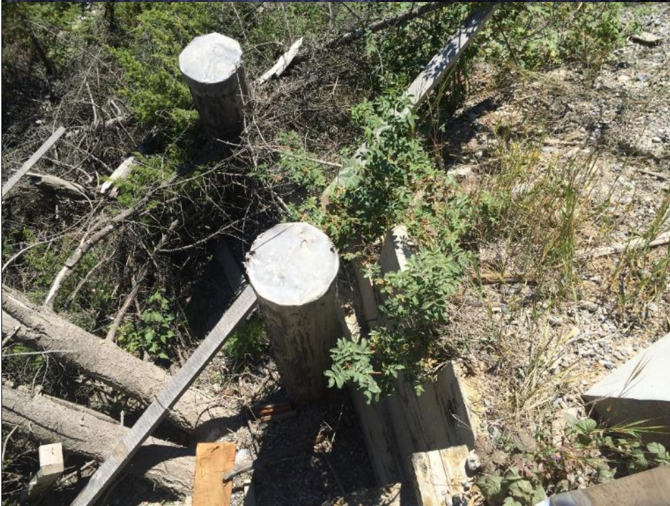
Photo #26 Abutment 2 - D.S wingwall
