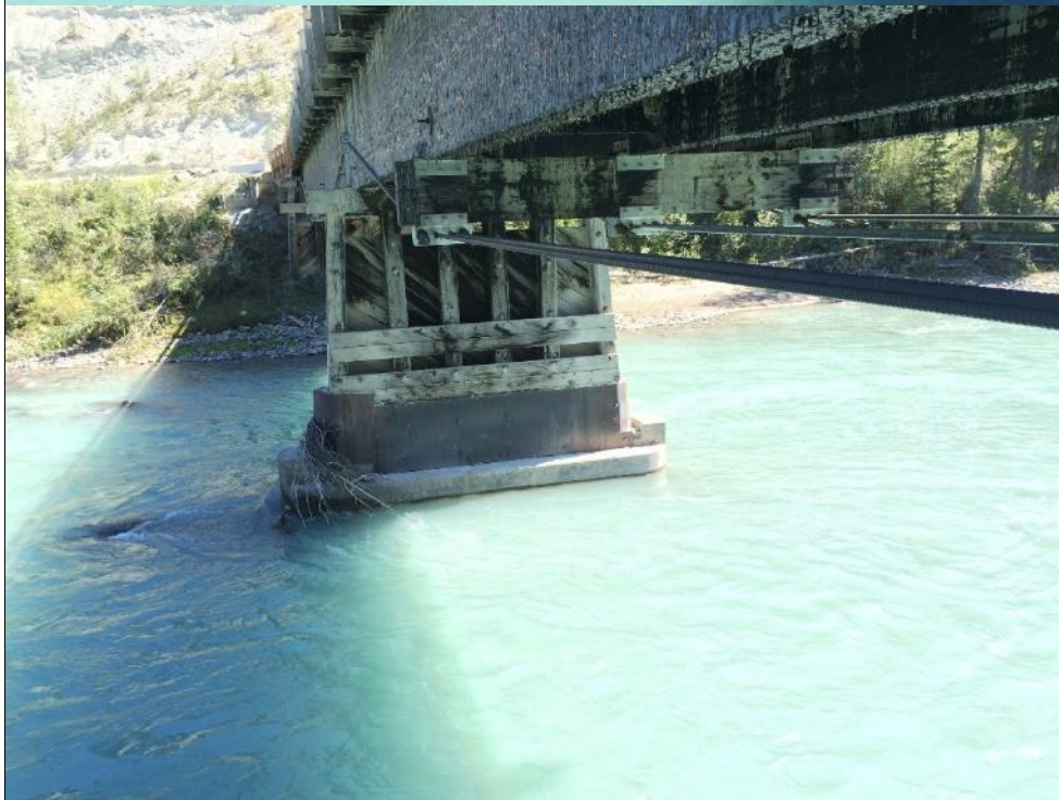
Photo #12 Pier 2 – looking to Abutment 1
