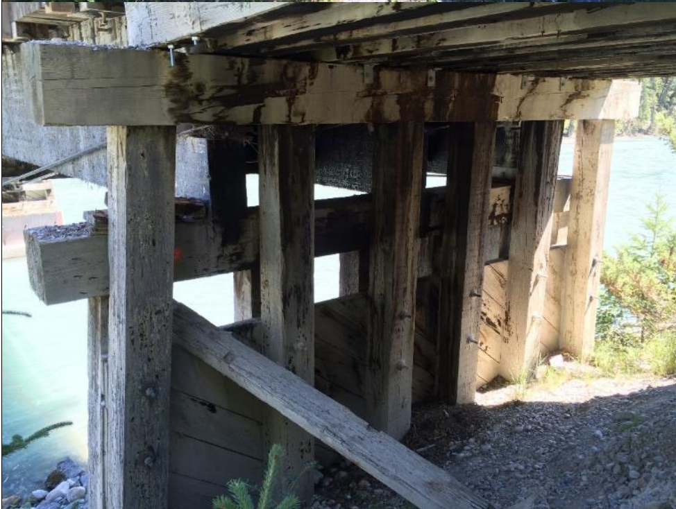
Photo #20 Pier 4 – looking to Abutment 1 / D.S
