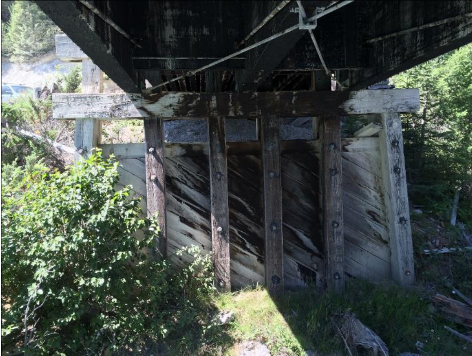
Photo #19 Pier 4 – looking to Abutment 2
