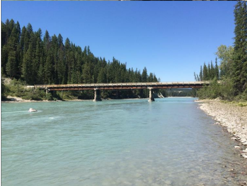
Photo #2 Downstream elevation
