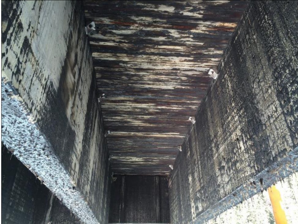
Photo #35 Interior faces of Girder 2 & 3
